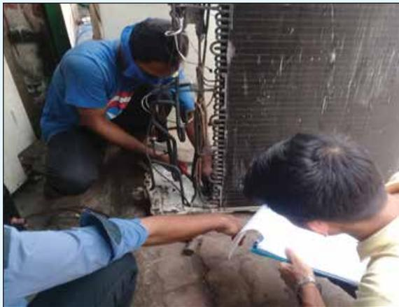
**Photo 5.2 (a): Worker with a Face Mask while Dismantling a Fridge.**
