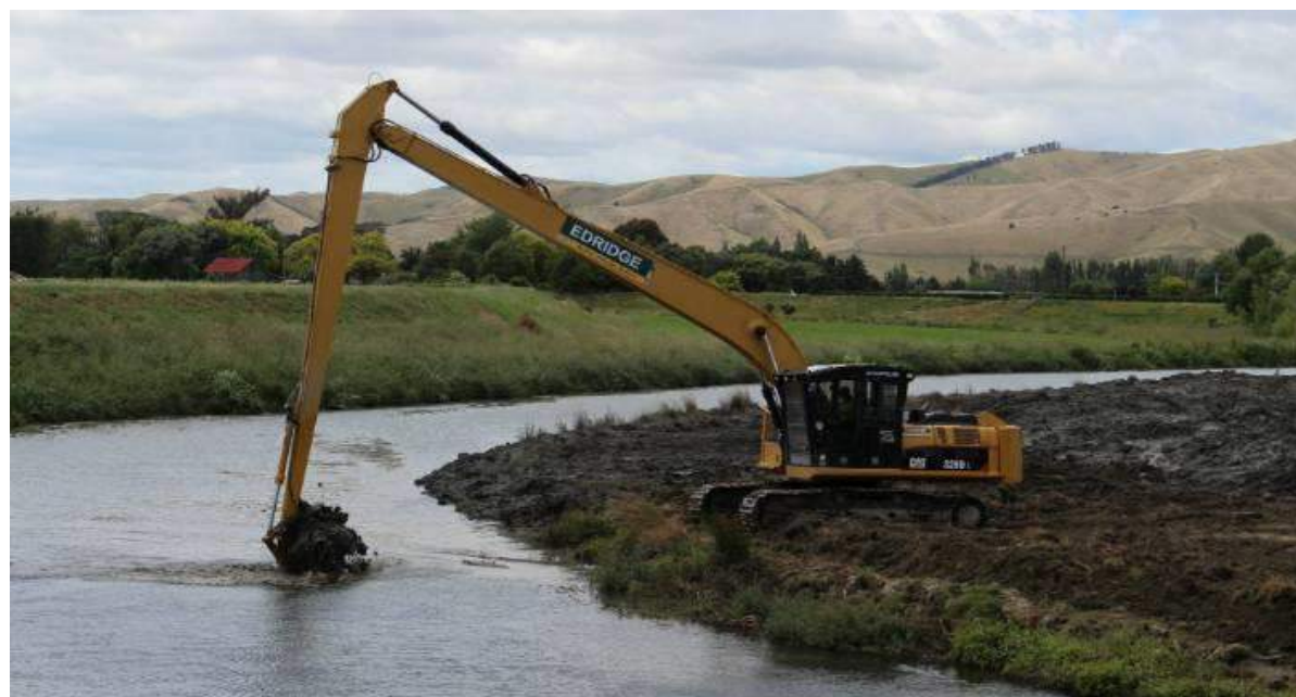
Figure 9.6: Image of River Sediment Dredging
