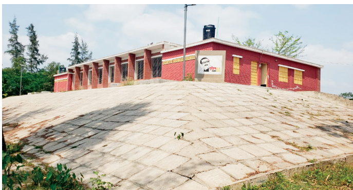
Mujib Killa specially designed raised land to provide shelter for people and livestock during the cyclone and tidal surge.
