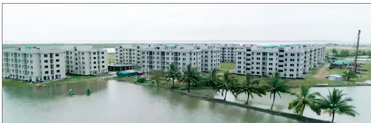
On 23 July 2020, Hon’ble Prime Minister Sheikh Hasina inaugurated 20 newly built special structures having 32 flats each with all amenities where 600 families get new shelter
